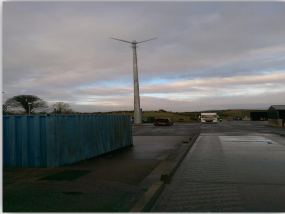
Wind Turbine Installation at Dungarvan CAS
