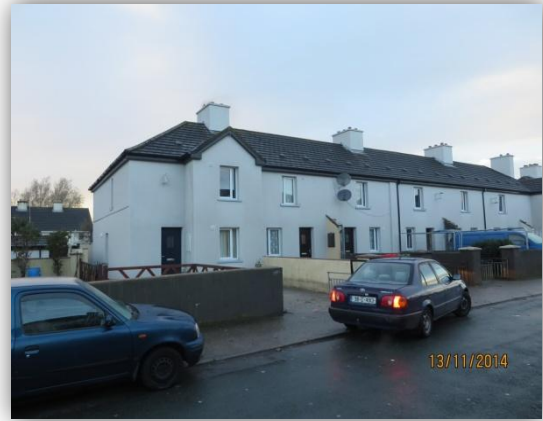
Housing Insulation Upgrade
